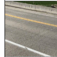
Roadside Abrasion in Wheel Paths
