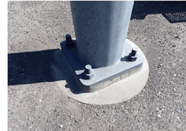
Base looking north.
